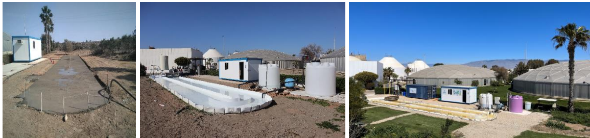
Figure 12: Evolution of the solar photo-Fenton plant
