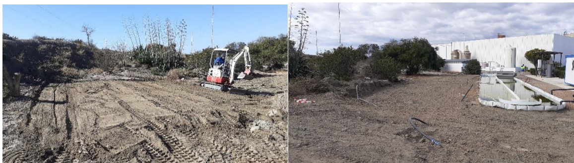
Figure 11. Construction works of the crop testing area
